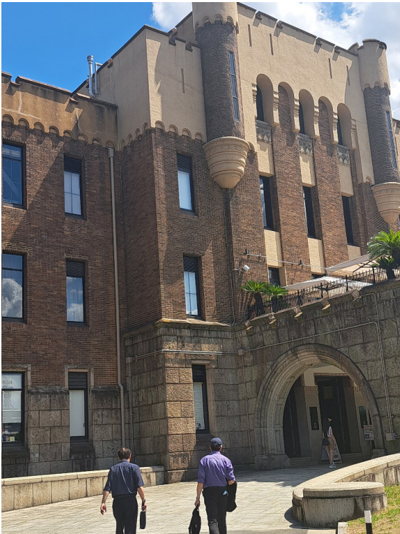
Photo A6. The building of the National Museum in Osaka [photo B. Piwowska].
