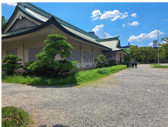
Photo 1. Shudokan building in Osaka [photo B. Piwowarska].
